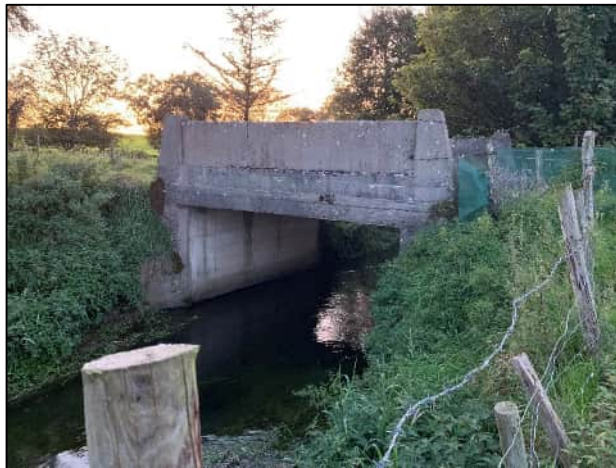
Plate 3-14: Concrete slab bridge with no suitability for roosting bats
