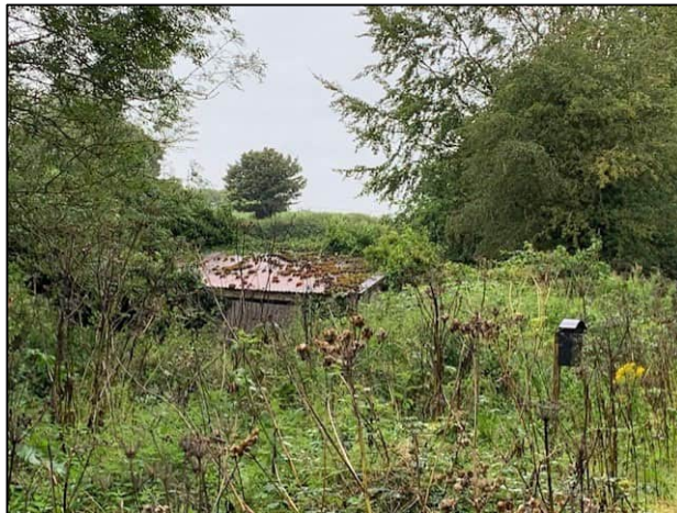
Plate 3-13: Small shed located at the north of the proposed site
