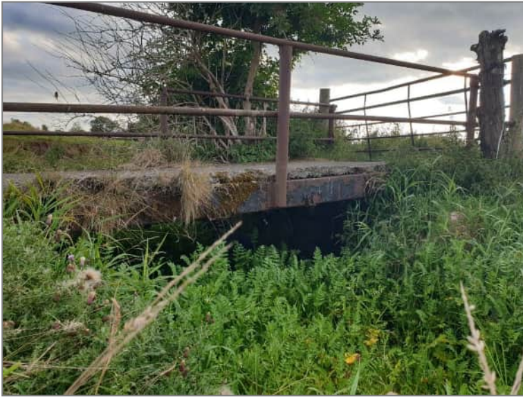
Plate 3. No bat signs and negligible roost suitability in this concrete bridge
