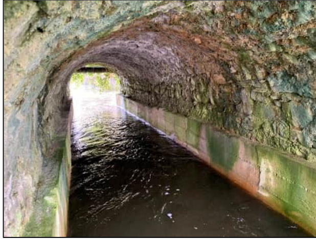
Plate 3-15: Masonry arch bridge on the southern boundary of the site with crevices suitable for roosting bats
