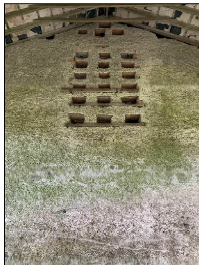
Plate 3-12: Recesses within the wall of the outbuilding with bat potential
