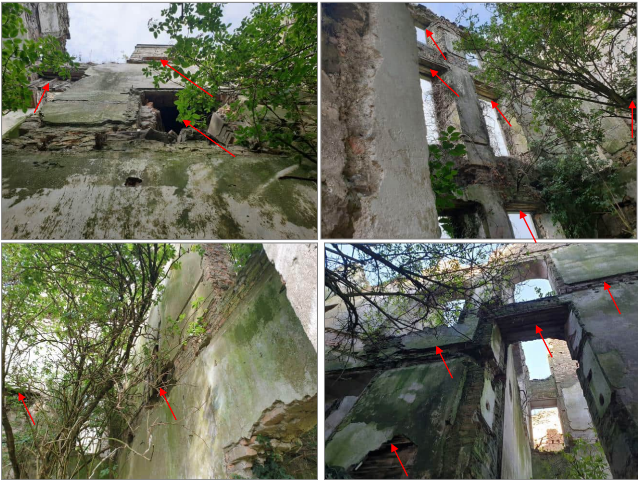
Plate 23. Rosmead House ruins; some examples of places where bats could find roost shelter during the day; open fireplaces and chimneys, space behind wall plaster and timber lathes, crevices above window and door lintels, cracks, hollows and crevices in stone and brickwork of walls
