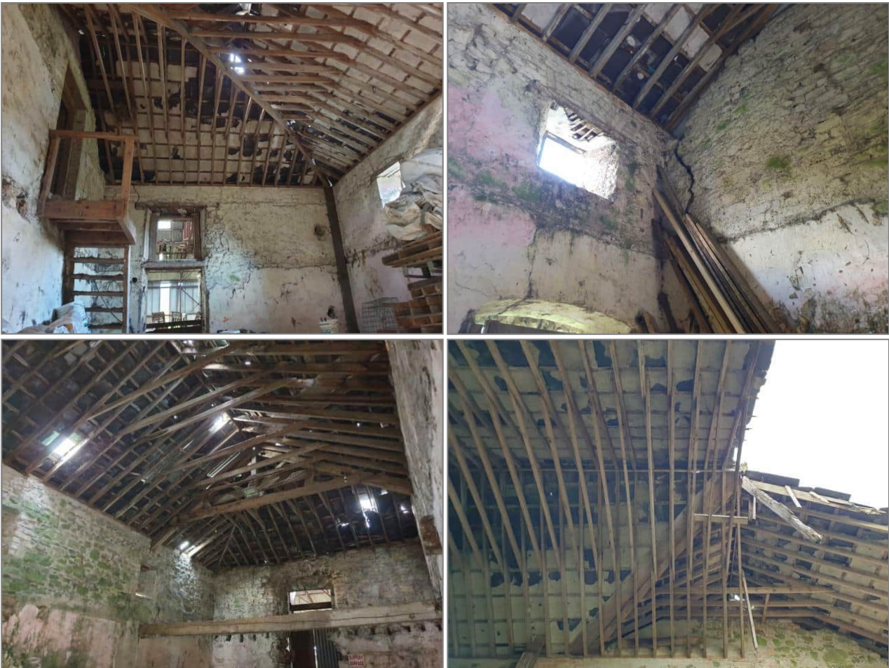
Plate 21. Examples of holes in the roofs of sheds in farm courtyard, also showing potential roost cracks and crevices
