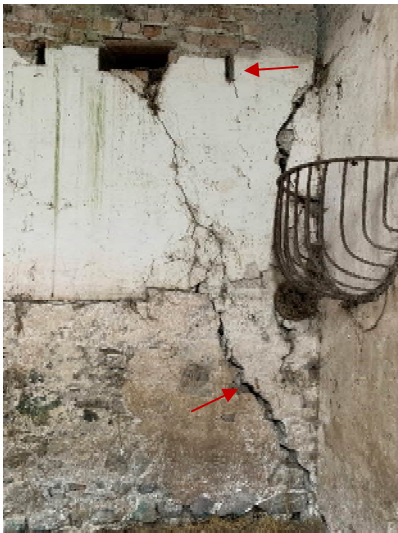
Plate 3-11: Potential roosting spaces in gaps and cracks within stonework
